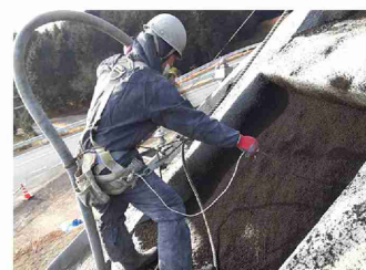
枠内植生基材吹付
