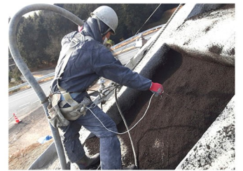
枠内植生基材吹付
